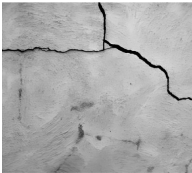
挡土墙裂缝
